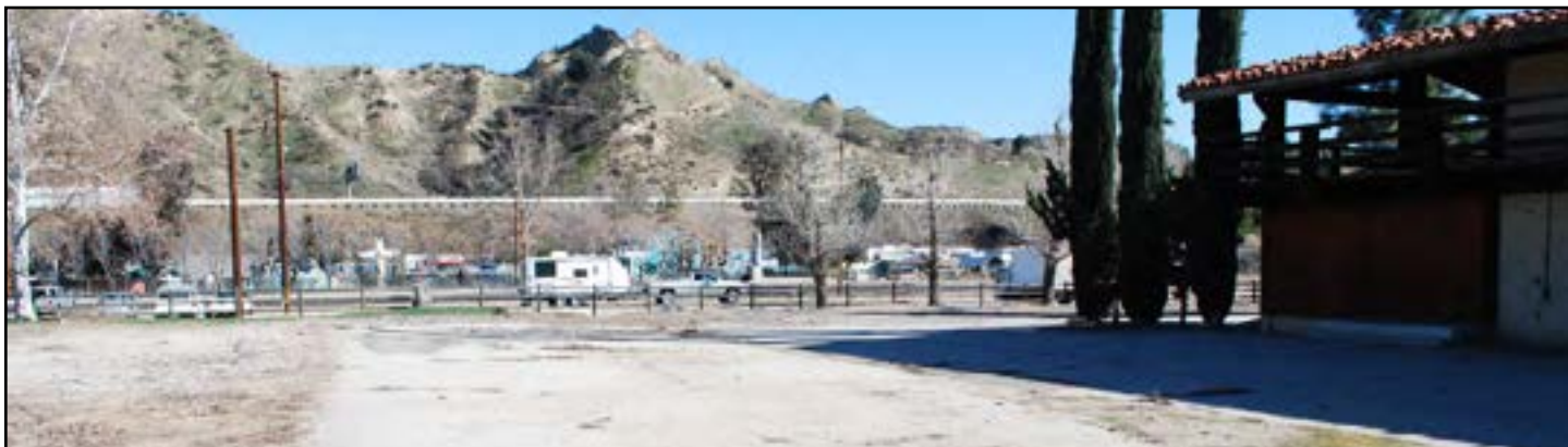
Existing lodge building and asphalt paving should be demolished.
